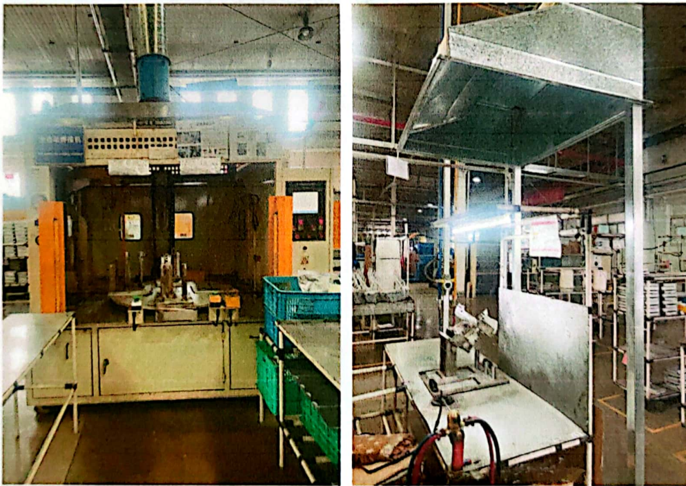
焊接工序集气管线和集气罩
